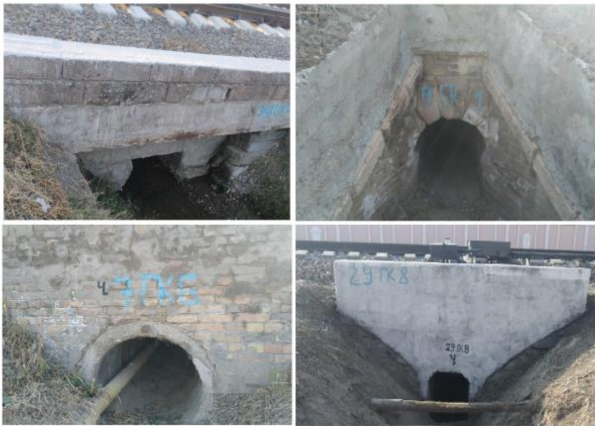
1- figure. The state of the waterproofing pipes located on the railway.
